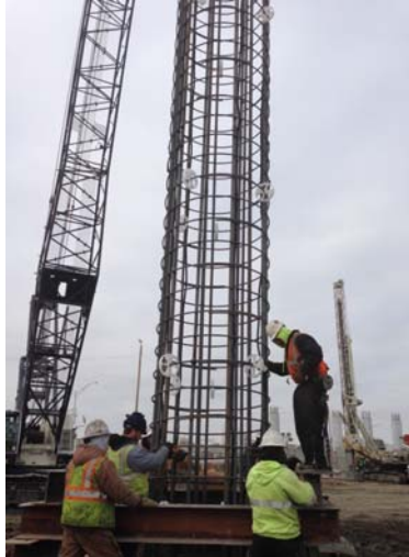
Setting up of cage with DYNA Force sensors in drilled hole
