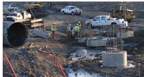
Completion of concrete pour of drilled shaft with DYNA Force sensors
