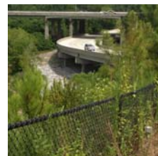
After adding new road
